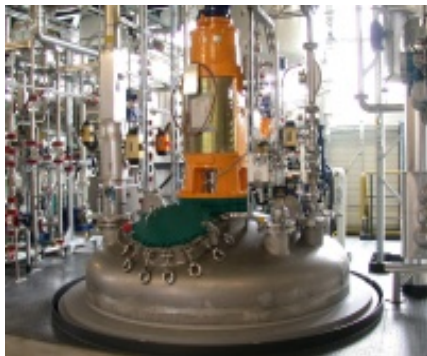
600 gallon stainless steel, jacketed, agitated reactor that we purchased and removed from site as part of the project
